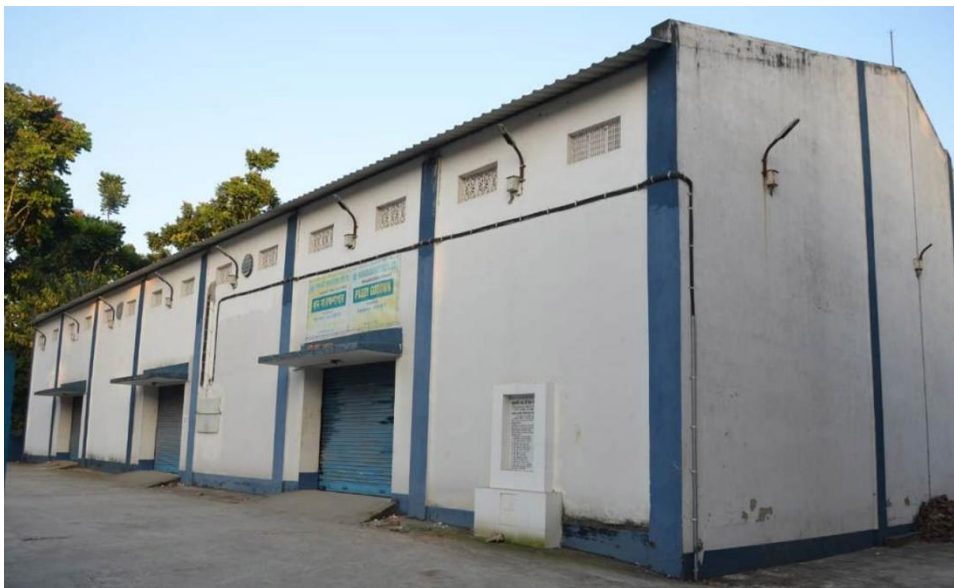
Figure 4: 1000 MT Godown built under RIDF
